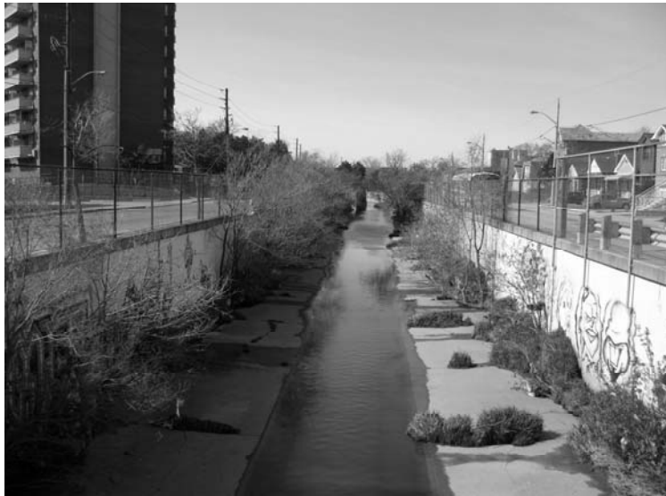
Existing condition of Black Creek at Humber Boulevard
