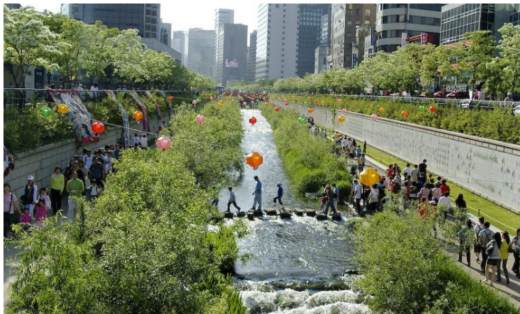
View of the restored Cheonggyecheon
